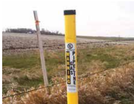
Landfill Gas Pipeline Marker
