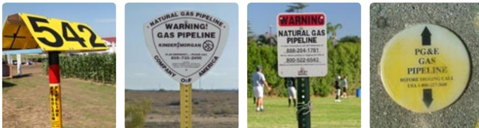
1. Markers include the name of the operator, the product in the pipeline or type of utility line and an emergency phone number.
